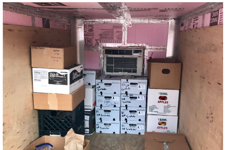
Photo 3.7. Interior of the mobile cooler with plywood floor and walls, XPS insulation, an A/C unit and taped sides.
