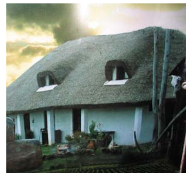
The guest house at BIO-Uruguay provides housing, dining, and meeting space for visitors.
